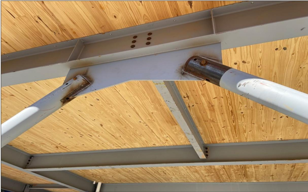
**Figure 3** Wood-steel hybrid structure (Tonelli, 2022).
