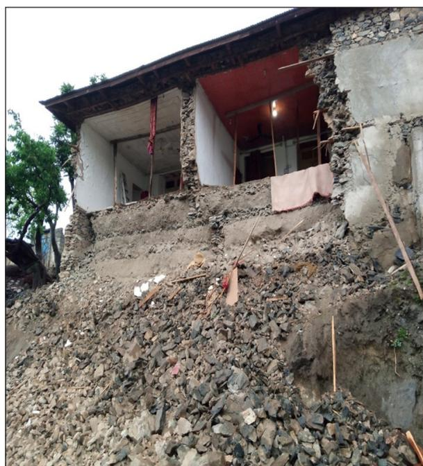
**Picture 13** Damage to House in Landslide.
