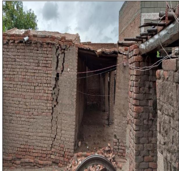
**Picture 4** Rain & Flood Damage.
