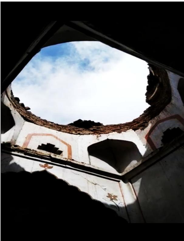
**Picture 7** Heavy Rains Collapsed Masonry Dome.
