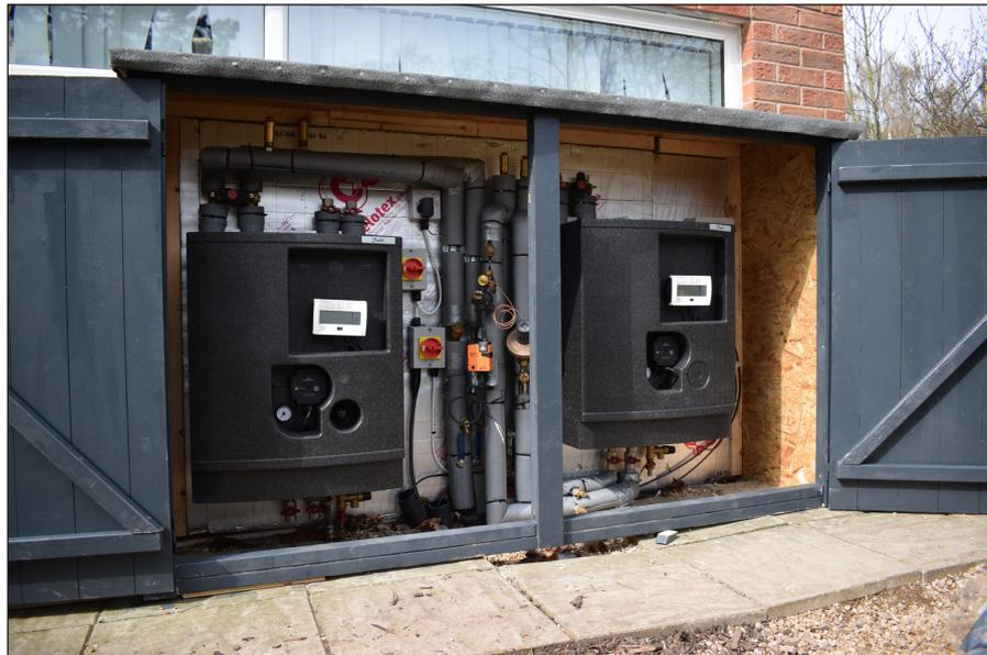
Figure 5: HIU in situ outside the Tarmac CdFH 4 house. Prosumer unit (right), consumer unit (left) (SAV systems, 2016).
