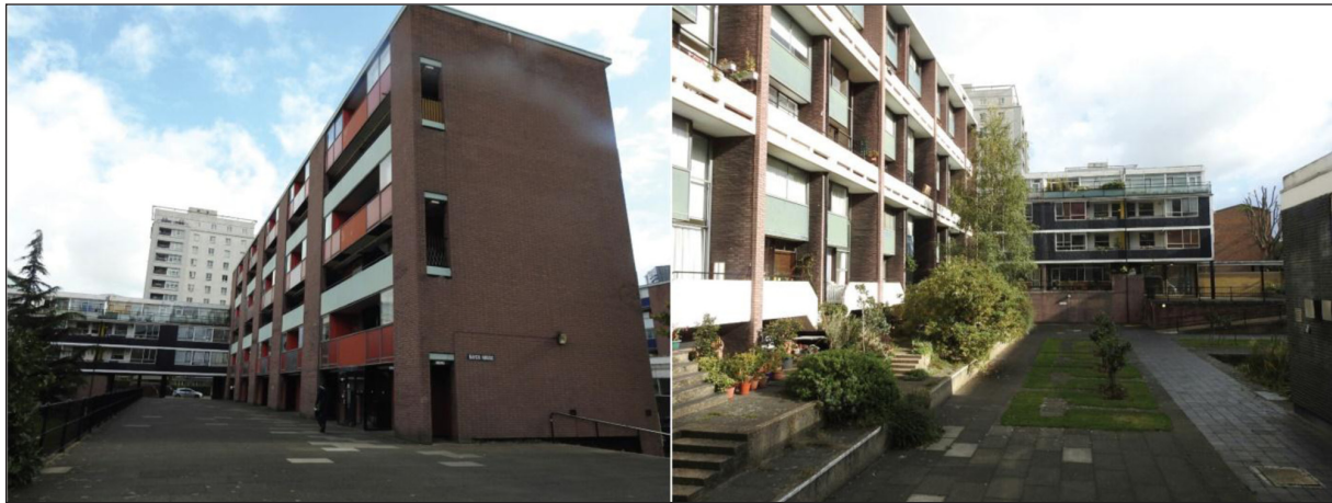
Figure 25: View of the Bayer house facing North (left) and facing South (right).
