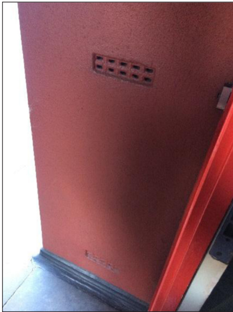
Figure 28: Airing brick on exterior wall.
