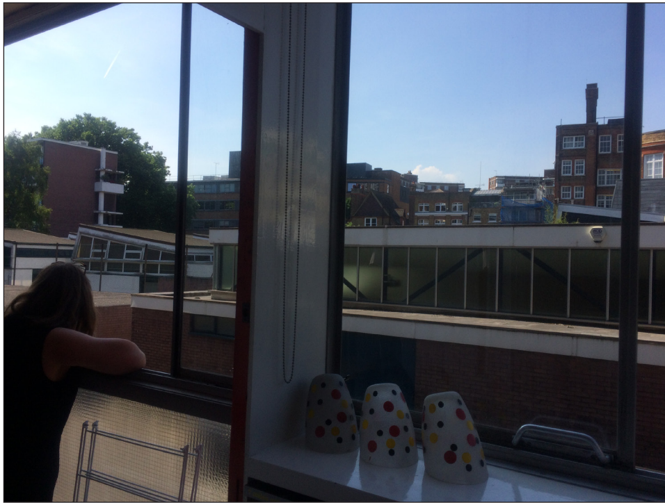
Figure 31: Single glazed window in North bedroom sliding from indoor to outdoor balcony.
