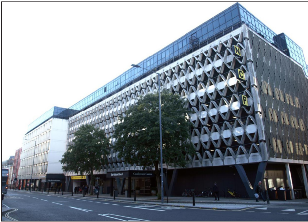
Figure 5: Kenneth Wakeford, Jarram & Harris Prince Street Car Park, Bristol, United Kingdom, Façade. Photo Szopinska-Mularz.
