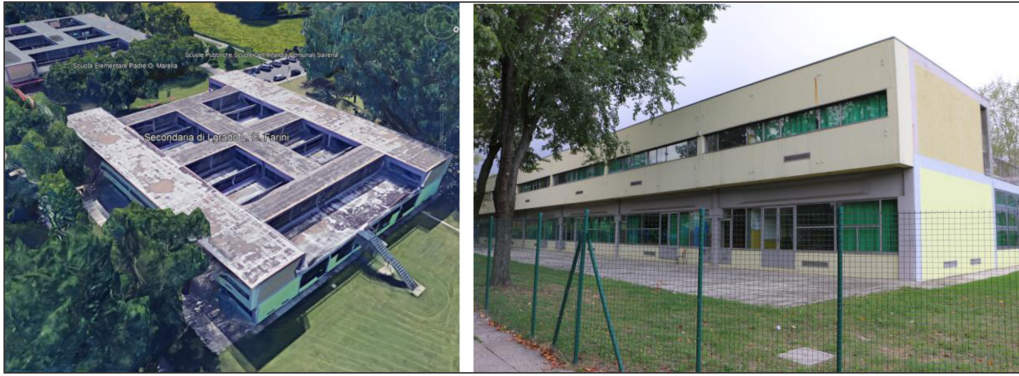
Figure 2: The elementary and secondary school L. C. Farini, built in 1975. Photo: Google Earth (left), a collaborator of the author (right).
