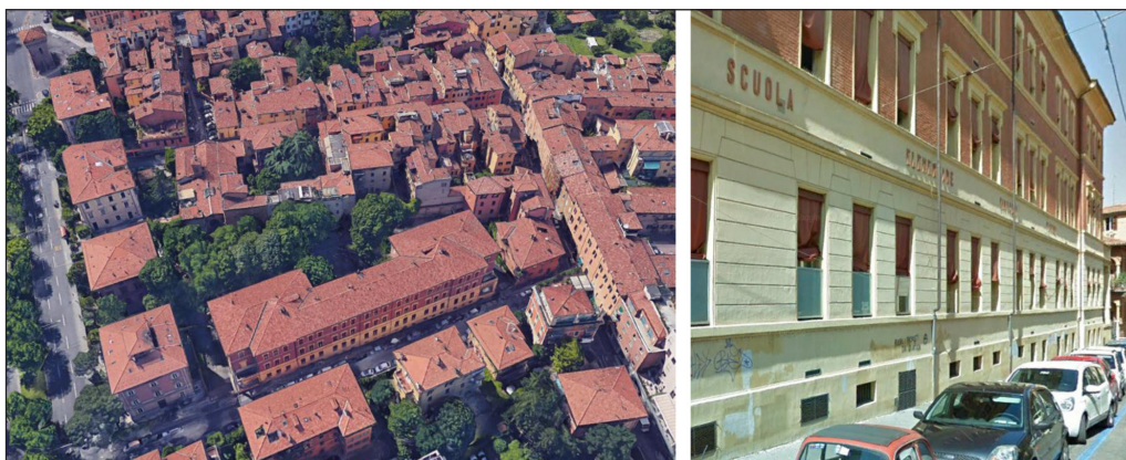
Figure 1: The elementary school G. Pascoli, the long building in the middle of the image on the left, built in 1915. Photo: Google Earth (left), Google Street View (right).
