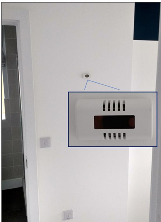
**Figure 1:** An EnOcean temperature and relative humidity sensor installed in one of the properties. A magnified view is shown in the inset image.
